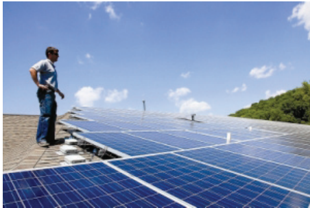
(Photo by Sara Hudock-Cole/New Jersey Herald) Todd Oekson of East Coast Alternative Energy in Sparta stands on the roof of the Goddard School, where his company installed 195 solar collection panels last year.
