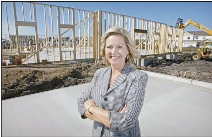
Marsha Bittner stands in front of the Goddard School under construction at 4665 44th Ave. S. in Fargo. The new state-of-the-art 8,400-square-foot building has been designed to accommodate approximately 140 children from infancy to 6 years old. The new school is projected to open this winter. David Samson / The Forum
